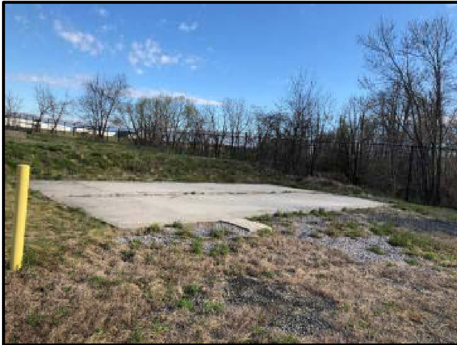
Photograph 1 – View of a concrete pad that held two above-ground fuel storage tanks at the NJ National Guard Area (East area), facing north.
